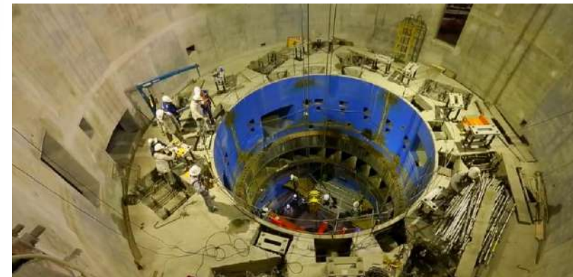
Civil Works at the Powerhouse: turbine's assembly
