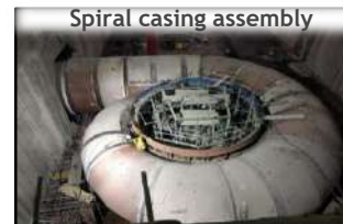
Spiral casing assembly
