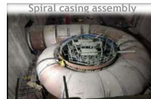
Spiral casing assembly
