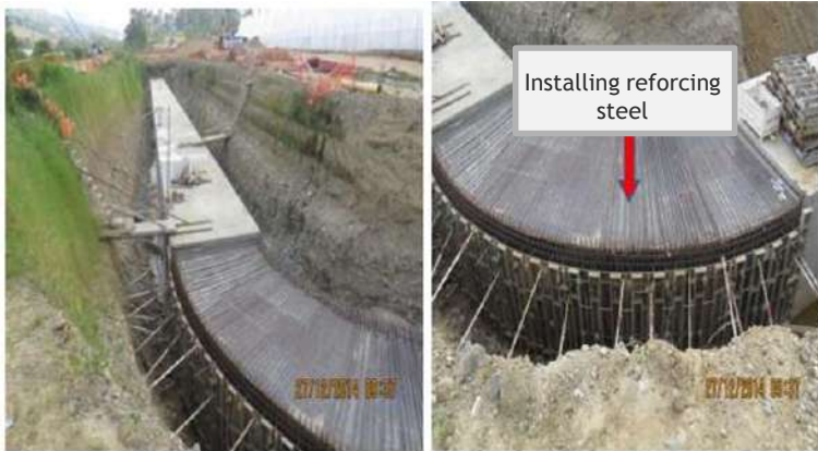
stretch of the discharge canal
